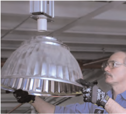
Remove metal reflector
